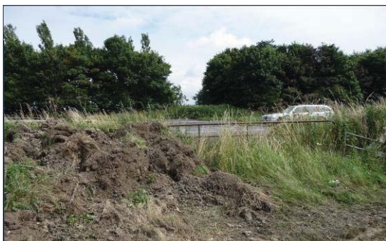
① Former at-grade carriageway crossing location
