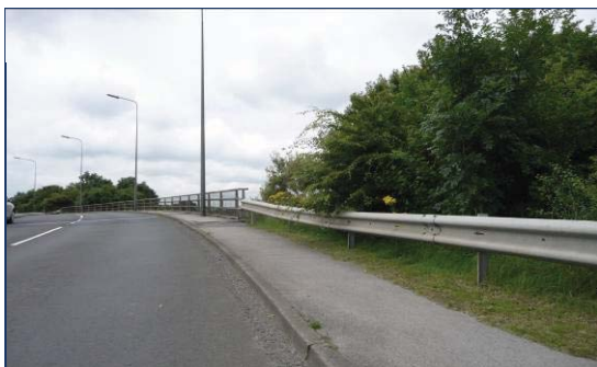
① Footway's eastern approach to overbridge
