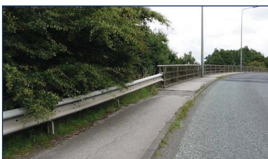
④ Footway's western approach to overbridge
