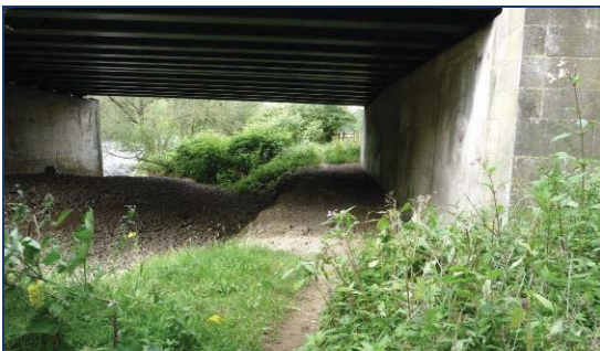
② Underpass below bridge carrying A1 over river
