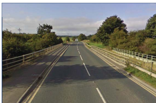
① A6136 Catterick Road overbridge
