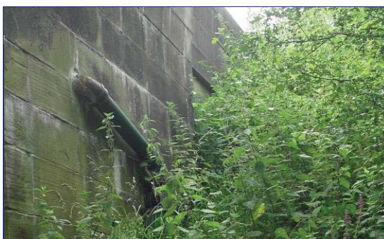
③ Embankment up onto A1 at western side of bridge
